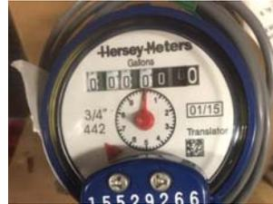
Most customers have a meter that looks like the meter here. The red triangle located at the bottom of the meter only moves when water is passing through. If you suspect you may have an issue, turn off all water inside and outside your home, locate your meter, and monitor the "red triangle". If the triangle is moving this indicates that water is passing through the meter.
